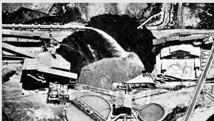
Figure 8.1.2. The subsidence sinkhole that engulfed the mine crusher plant in 1962.
