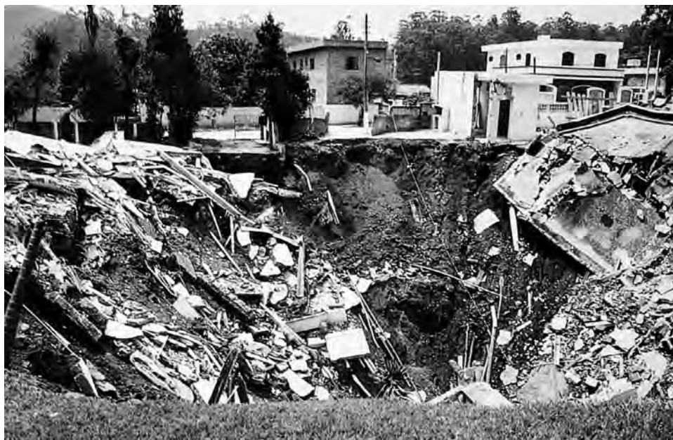
Figure 8.7. Collapse of a house in Cajamar, Brazil, in 1986 over a sinkhole induced in a thick soil cover by excessive groundwater abstraction at a nearby industrial site.
